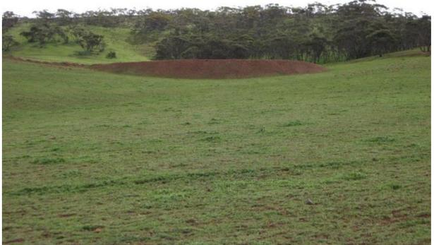
Hillside dams can provide a gravity-fed supply and use diversion drains to expand the catchment. The diversion drains (or banks) also protect the downslope paddocks from soil erosion.
