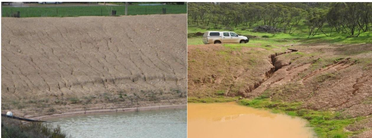
**Figure 16. Examples of rill and gully erosion on dam walls and inlets. Dispersive clays can hold water well but are highly erodible if flows are concentrated and soil surfaces are unprotected. (Figure 25 shows some options to control the risk of erosion on dam inlets and walls.)**
