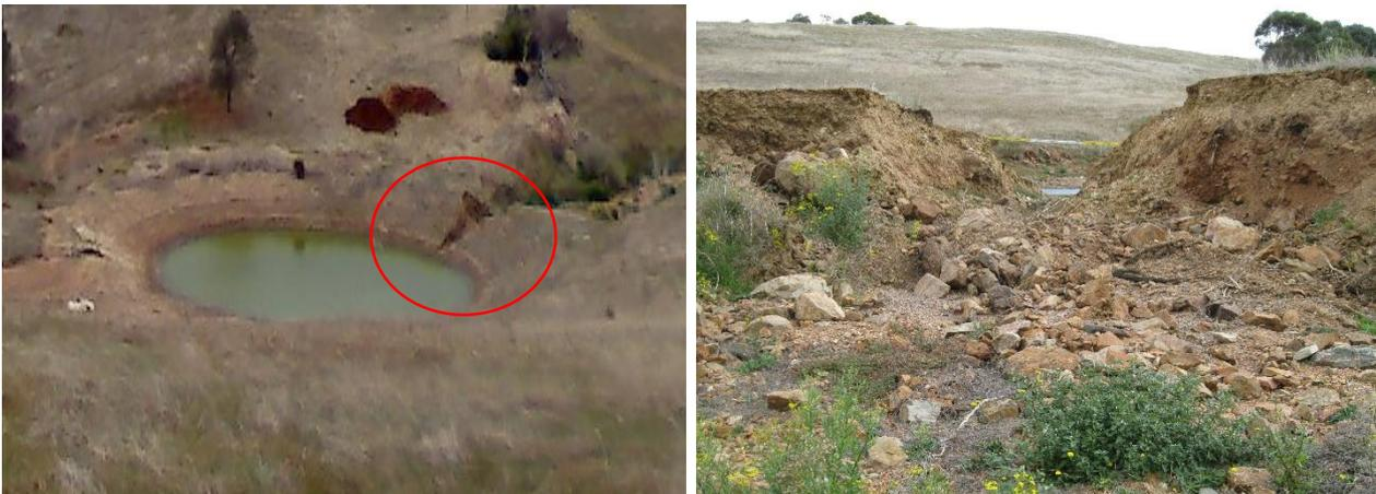
**Figure 41a. Examples of dam wall failure and washout due to inadequate spillway design and lack of sufficient freeboard.** Photos Dave Cunningham (L) & Seb Drewer (R)
