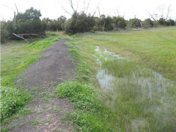
Well grassed diversion drains reduce the risk of erosion and further sediment entering the dam
