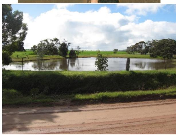
Off-stream dams sited adjacent to roads can take advantage of reliable runoff events from the bare, compacted road (which acts as a catchment).
