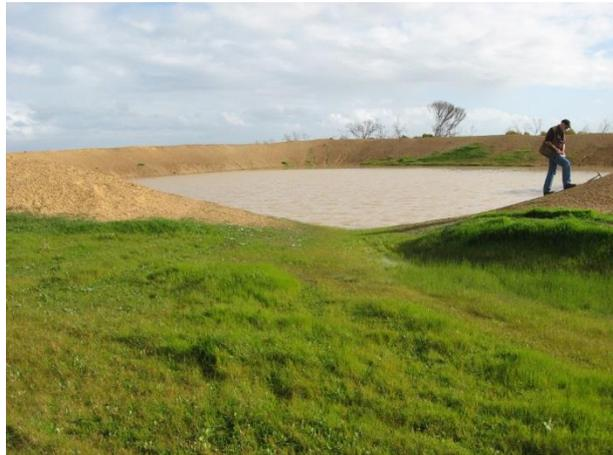
Maintenance of grass cover can protect the diversion drain and dam inlet.
