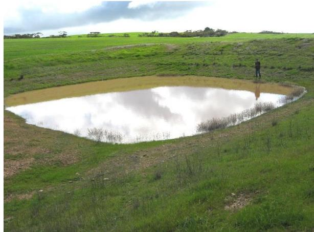
Excavated earthen tanks, sited in relatively low parts of the landscape are a common form of farm storage on EP. New dams of this type need to factor in reduced runoff rates from no-till farming practices to ensure sufficient catchment area.
