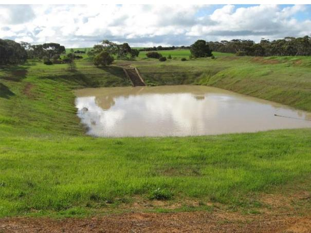
A concrete structure provides protection from inlet erosion, but at high cost.
