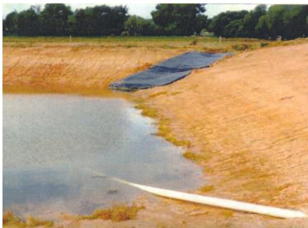
Cheap plastic sheeting also provides effective protection from inlet erosion.
