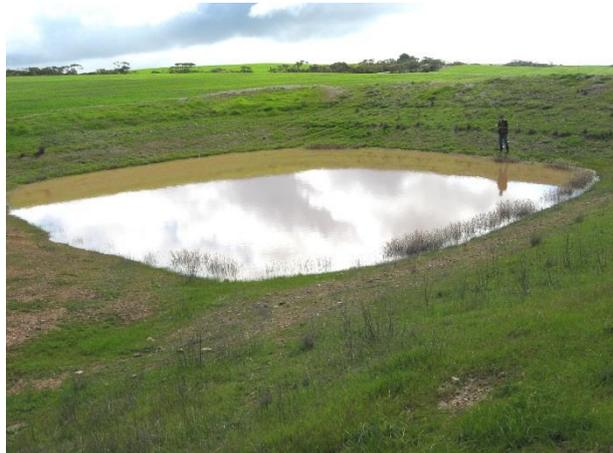
Spreading topsoil and establishing grass can be another cost-effective way to protect dam walls.
