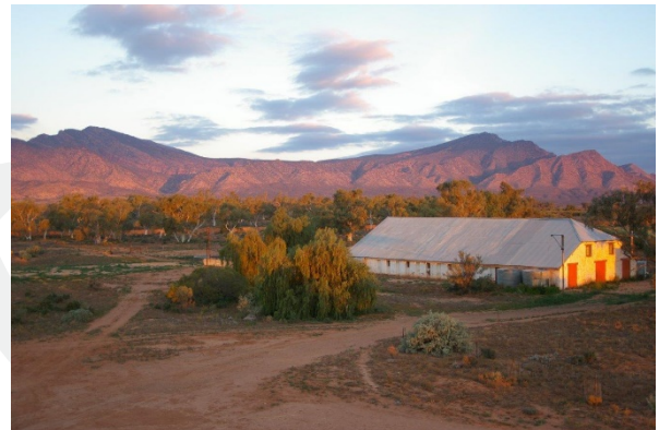
Edeowie Station Shearing Shed. Photo courtesy www.edeowiestation.com.au
