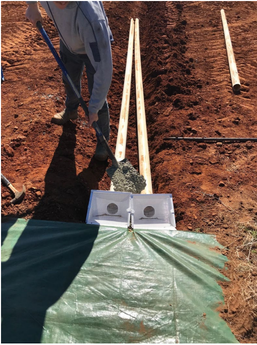
Installing the sump
