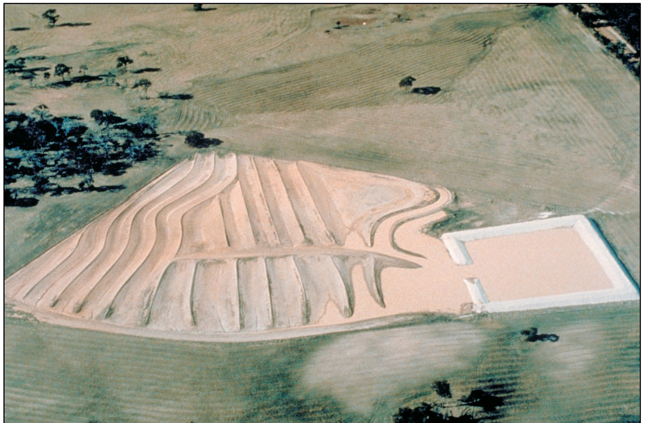
Figure 9: Roded catchment in WA with dam filled with water.
