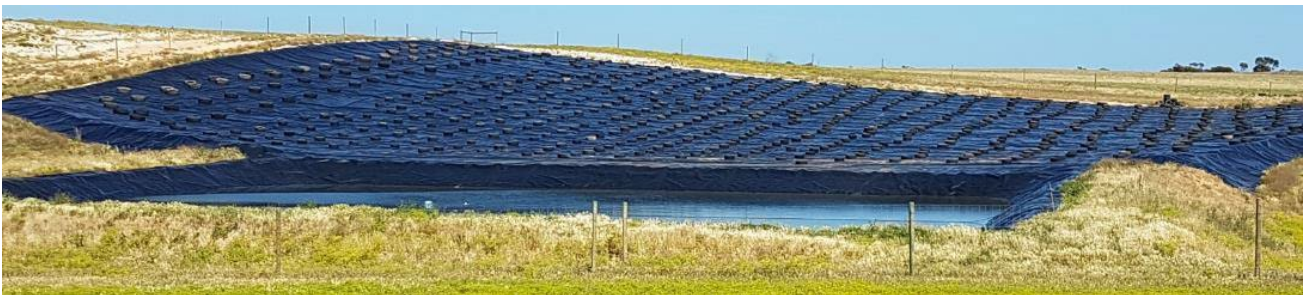
Figure 10: Sheeted catchment at Wharminda
