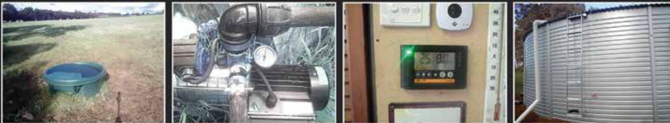
Caught on camera: Remote cameras can be put to all sorts of uses around the farm, from (left to right) checking stock watering points, monitoring pump water pressure, checking electric fence voltage, and tank water level.
